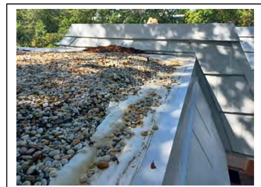
Pool building tar/gravel and edges with sealant
