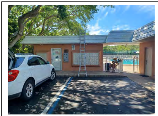
View at front of building
